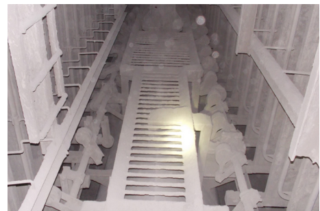
Internal ESP parts
